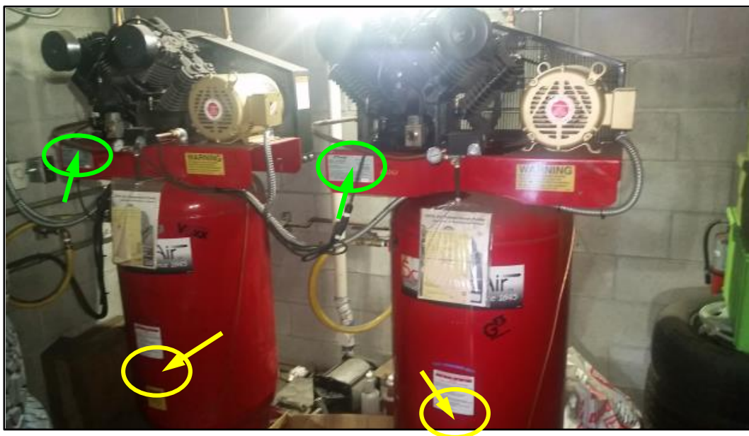
Figure 1. Location of the sticker with serial number information – green arrows and circles. Location of the nameplate on air compressor tanks – yellow arrows and circles.
